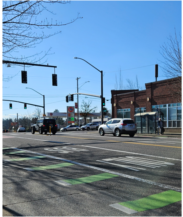
FIGURE 8. SW CAPITOL HWY & SW SUNSET BLVD TRANSIT STOP
